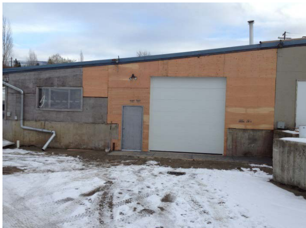
Remedial work new permit
